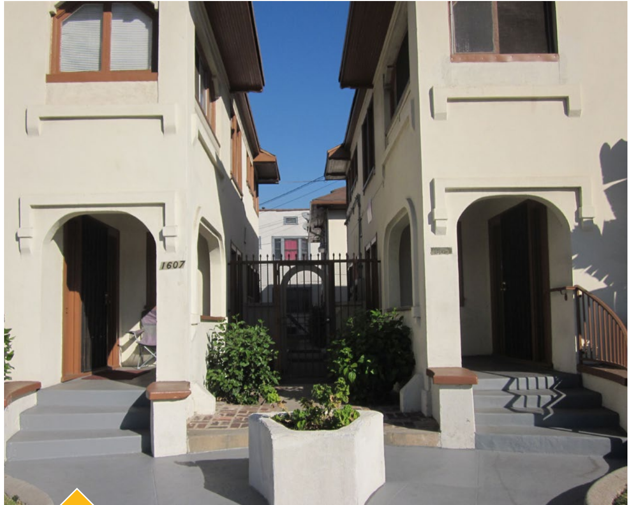
An example of a well-designed multi-family complex (Martin Luther King & Harvard). The re:code LA project provides an excellent opportunity to ensure that new multi-family can achieve a higher quality of development.
