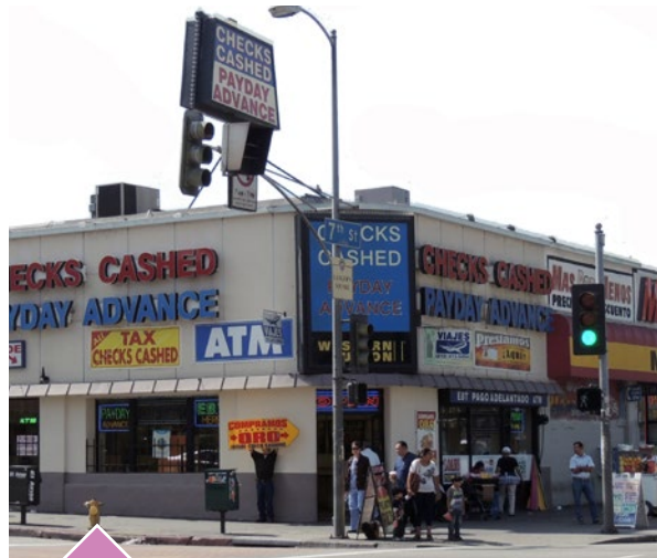
A clutter of temporary signs actually reduce the effectiveness of other signs on the site.
