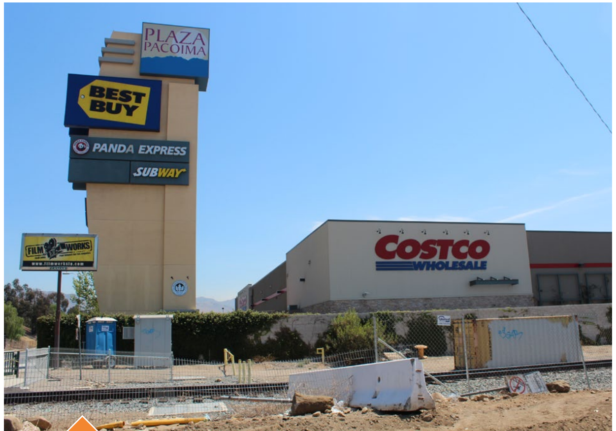
This recently-built shopping center is a redevelopment of a former manufacturing facility and is a prime example of the conversion of industrial land to a higher-performing retail use.
